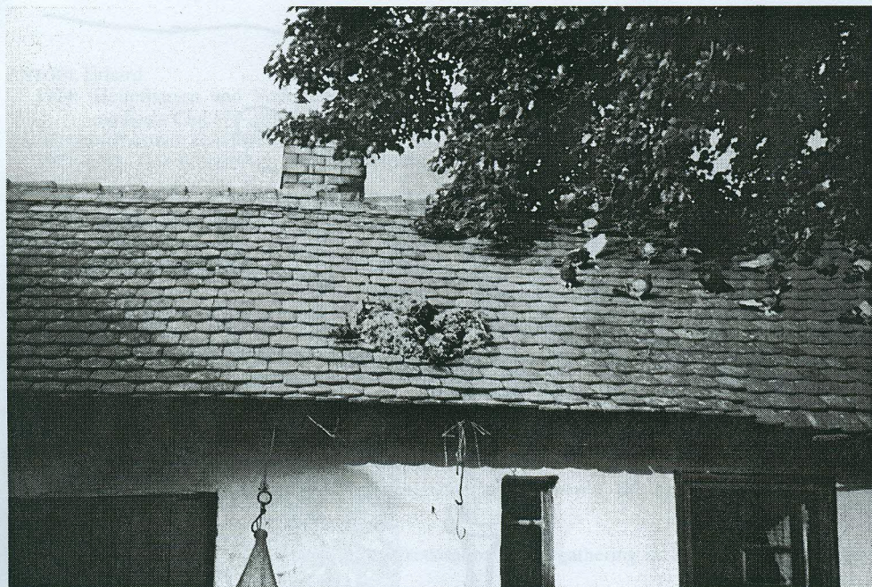
Fig. 3. Sempervivum on the roof of a farm-house (Domaszék, S-Hungary)
